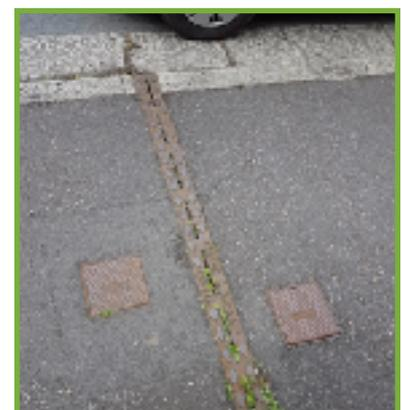
An example of this is in Exeter, where an EV owner has been permitted by Devon County Council to install a buried duct within the footway to temporarily accommodate a cable to the car when needed, providing it is installed by an accredited contractor at the owners expense<sup>[20]</sup>.
